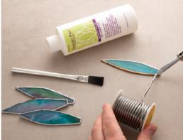
**STEP 4:** Hold two leaves together with just bottom edges touching and solder along joint. Repeat with remaining leaves (connect them one by one and work out from middle).
